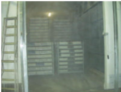
Figur 57: Innfrysingstunnel
